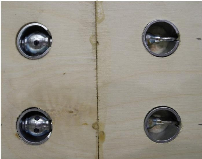
A stop plate was installed on each end of the board. These are necessary for positioning the scales and javelins.
